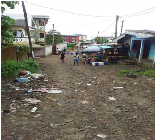
Photo 3 : Route of obstructed access by small businesses
