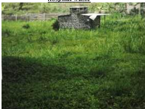
Photo 7 : Incinerator of the Buea Hospital unused and abandoned
