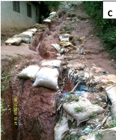
Photograph (A) shows the bed of a permanent, stable runoff stream. The photograph (B), presents a disorganized bed erosion factor and destruction of the slope. Finally, the photograph (C) shows an undeveloped road, destroyed by the diffuse runoff of rainwater in the absence of a gutter.
