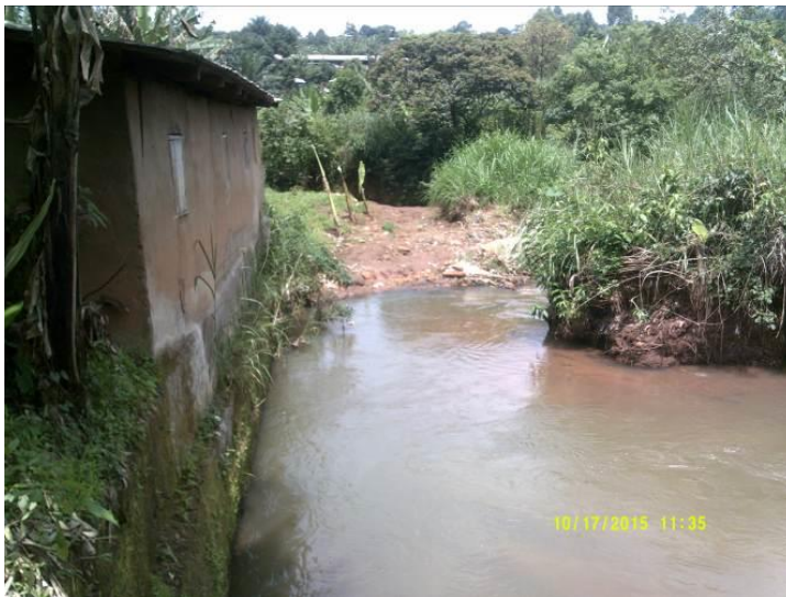
Photo 2: Example of construction at the edge of a watercourse
