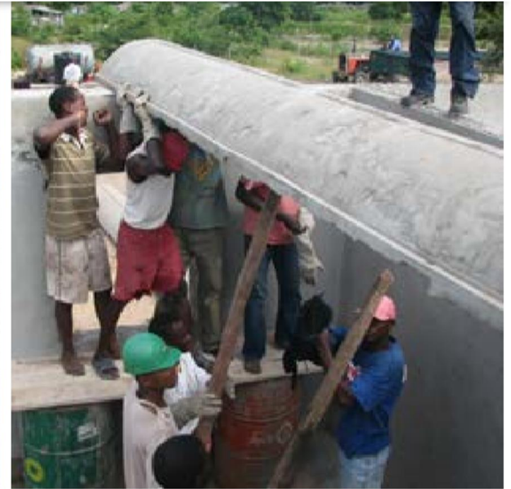
Participatory Prefabrication Process of Roofing Elements / Source: UN-Habitat
